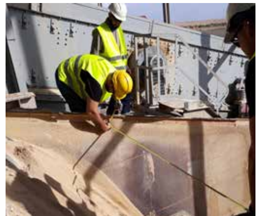
The project providing for the replacement of a 300 t/h screen for a phosphate installation, OCP SA, Morocco
